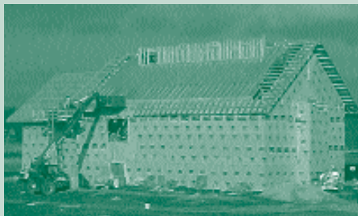
Hurstville Interpretive Center in progress.
