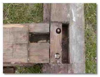
(picture courtesy of Trillium Del Timberworks) This is an example of a mortise and tenon joint that is 172 years old.
