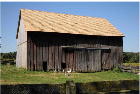
A historic 1842 barn outside of St. Charles, IL is undergoing a transformative restoration back to its original floor plan! Work began last month by lifting the structure, and pouring a new foundation...
